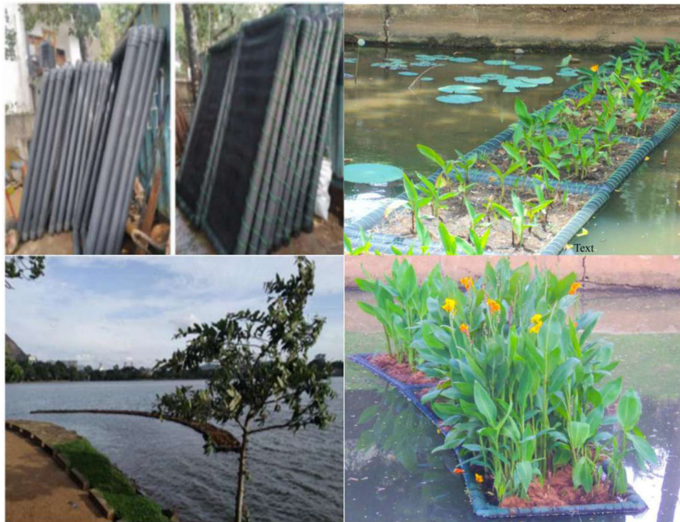
EXHIBIT 3 Implementation of floating wetlands in Kurunegala Lake. [Color figure can be viewed at wileyonlinelibrary.com ]
